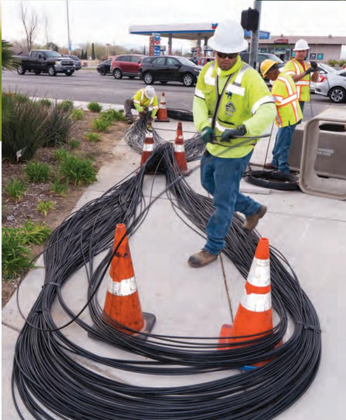
**"This advanced traffic management system is replacing legacy controllers, which have been in service for years and lack the sophistication of modern computerized systems. The new signals will communicate via high-speed fiber optic cables and coordinate their actions with neighboring signals, even across city boundaries."**
